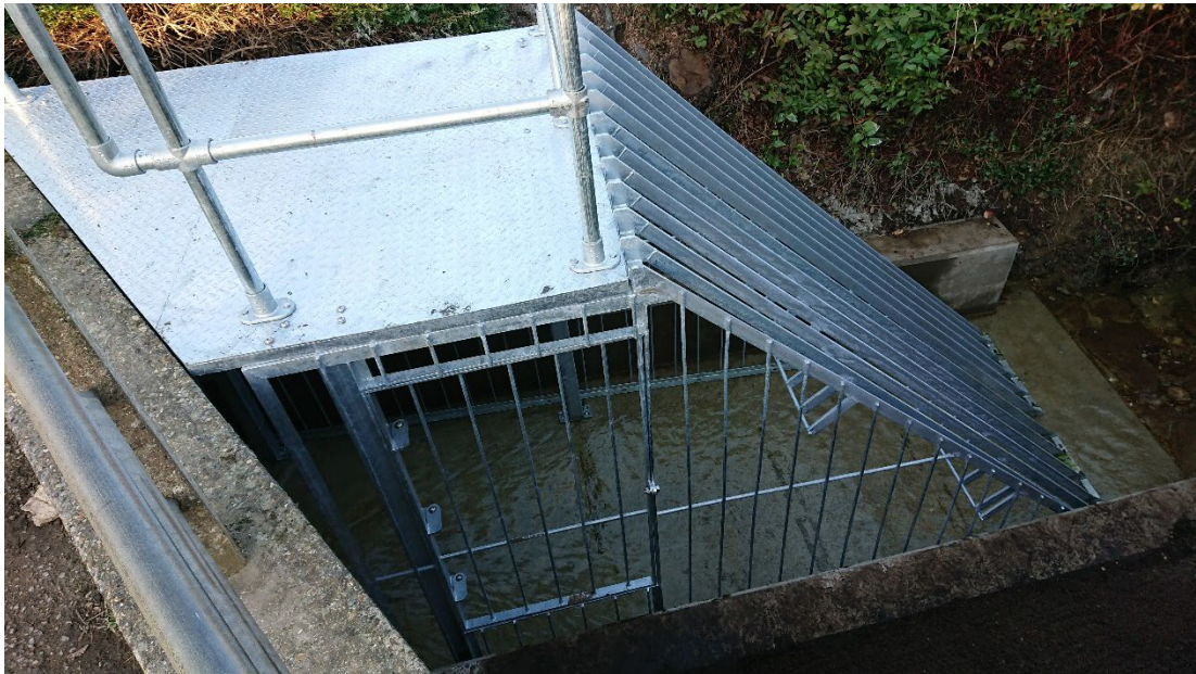
New Trash Screen at Mill Lane
